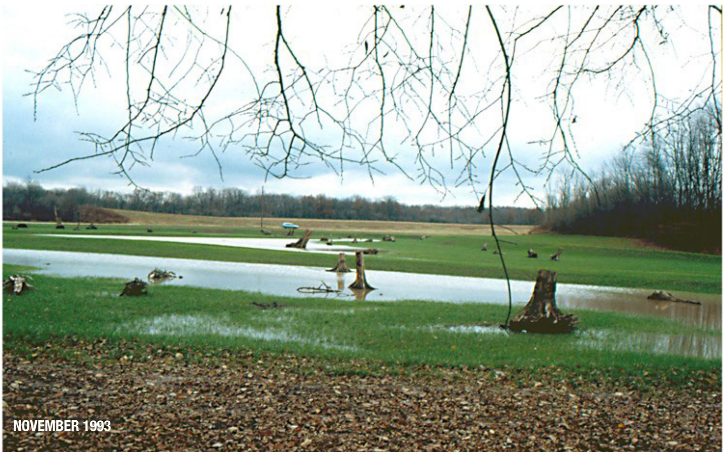
FIGURE 6. Following finish grading, stumps and other woody debris were placed to create escape cover for amphibians and singing/sentry platforms for various birds. The final task prior to onset of winter conditions was to protect the wetland from erosion. A combination of oats and annual ryegrass was seeded to provide rapid cover of the site. Effective as protective cover, these grasses did not compete with colonizing hydrophytes and soon succumbed to inundation. Yet, remnant stems and leaves acted to catch and hold “seed rain” from spring flooding in 1994 and to add detrital organic matter and nutrients to the soil substrate.
