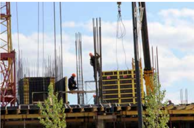
New construction in Astana (Kazakhstan) Photo: Shynar Jetpissova/World Bank
